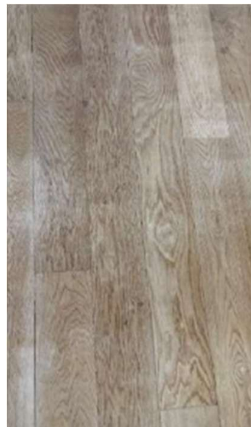
© RENOLAB.B project 070_Mundo B
