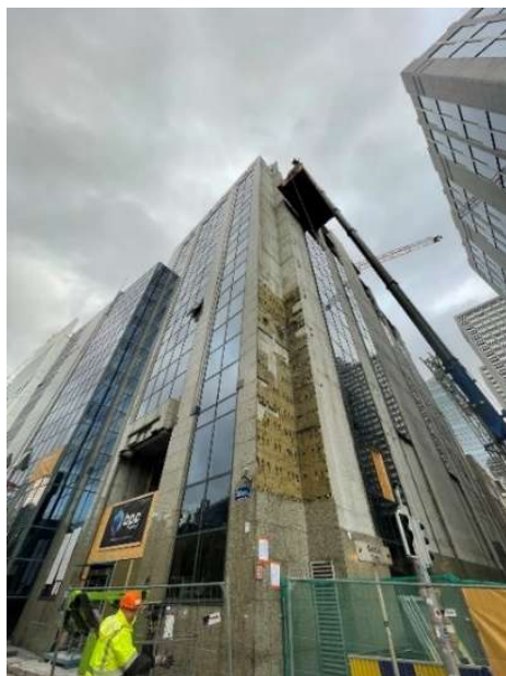
© RENOLAB.B project 097_NOR5
