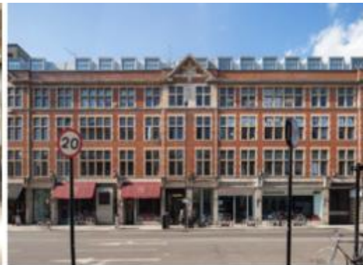
Refurbishment & Fit-out Homes & Commercial Buildings
