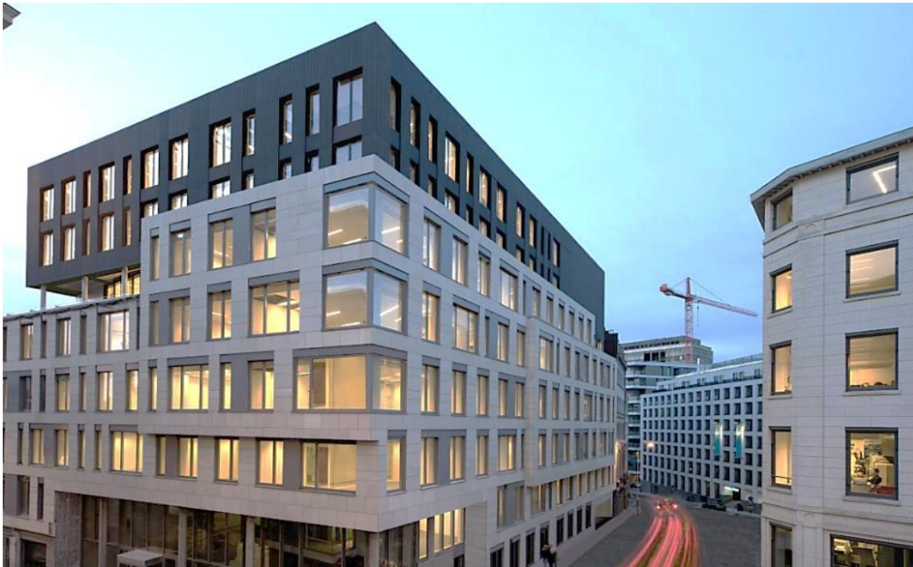
Project Treurenberg Brussel – Axa – Assar Architects
