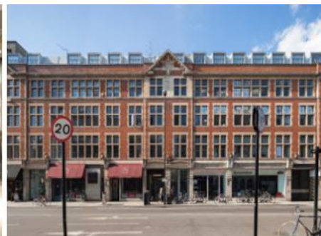
Refurbishment & Fit-out Homes & Commercial Buildings
