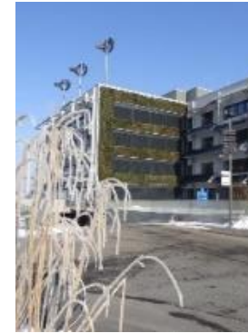
Solarwind Luxembourg Source: boydens engineering part of sweco
