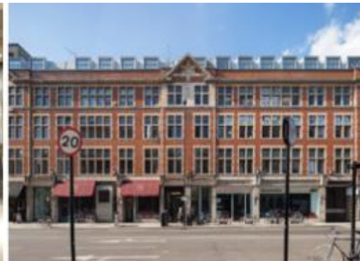
Refurbishment & Fit-out Homes & Commercial Buildings
